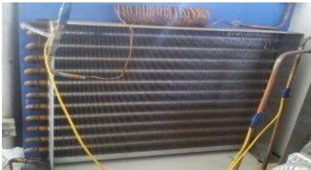
Fig.5 Fin Tube evaporator
