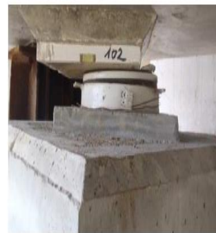
Fig. Bearing positions
